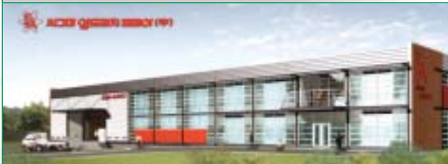
New facilities, like this $7 million warehouse in Korea, ensure rapid delivery of Life Science and High Technology products to customers.
