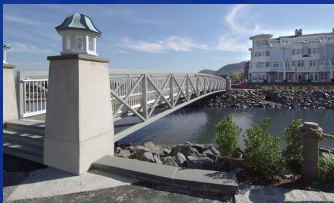
Harbors at Haverstraw development in Rockland County
