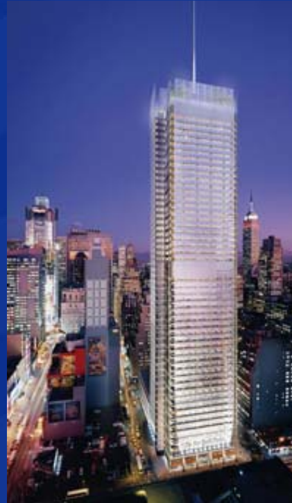
The New York Times Building Times Square
