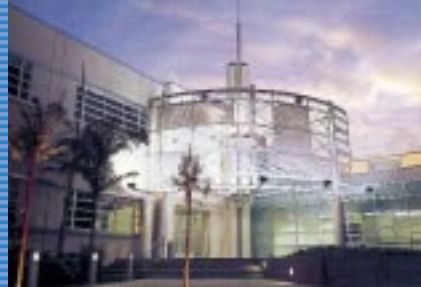
Westside Media Center
