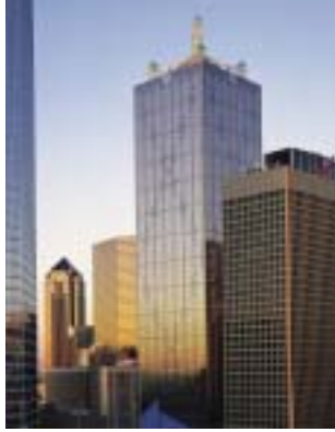
RENAISSANCE TOWER Dallas, TX
