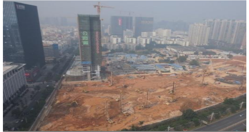
Excavation and shoring system in progress
