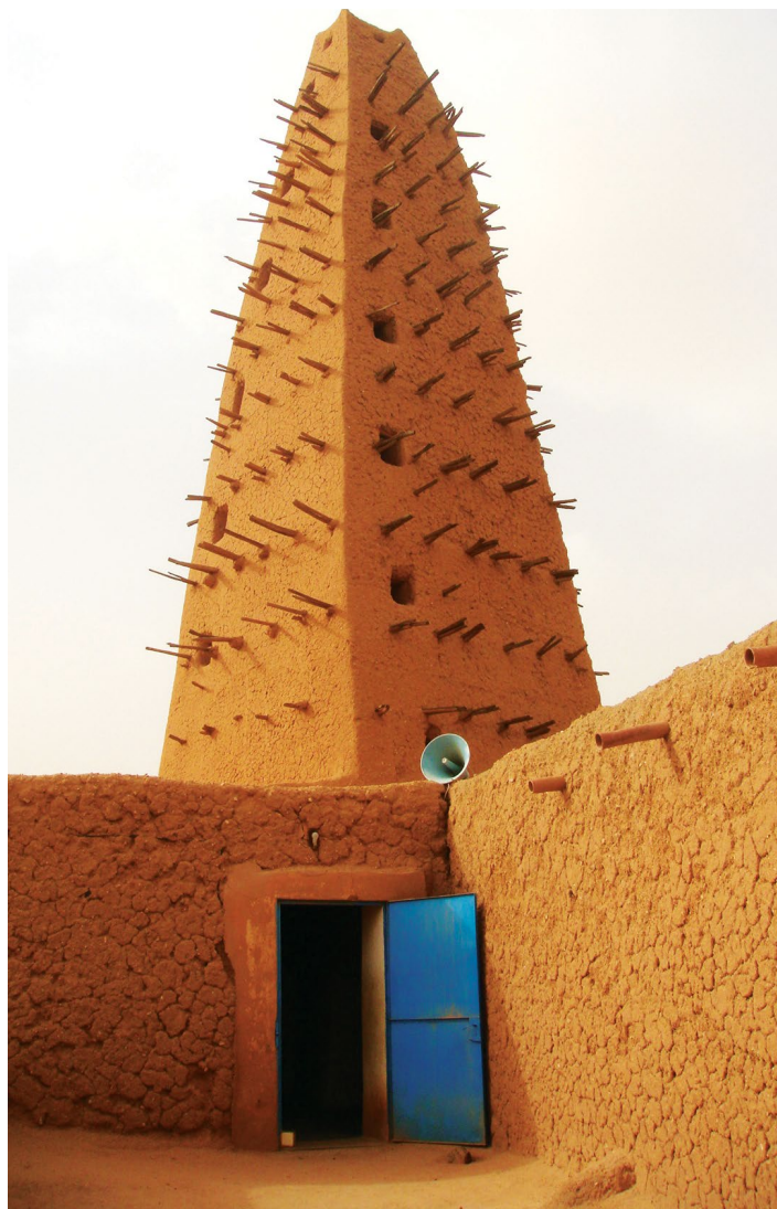
The Agadez Grand mosque. Made of clay, it was originally built in 1515 and restored in 1844.
